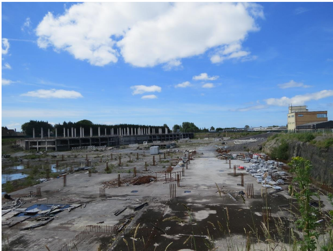
Image 4: Foundations built prior to project being abandoned in 2008
