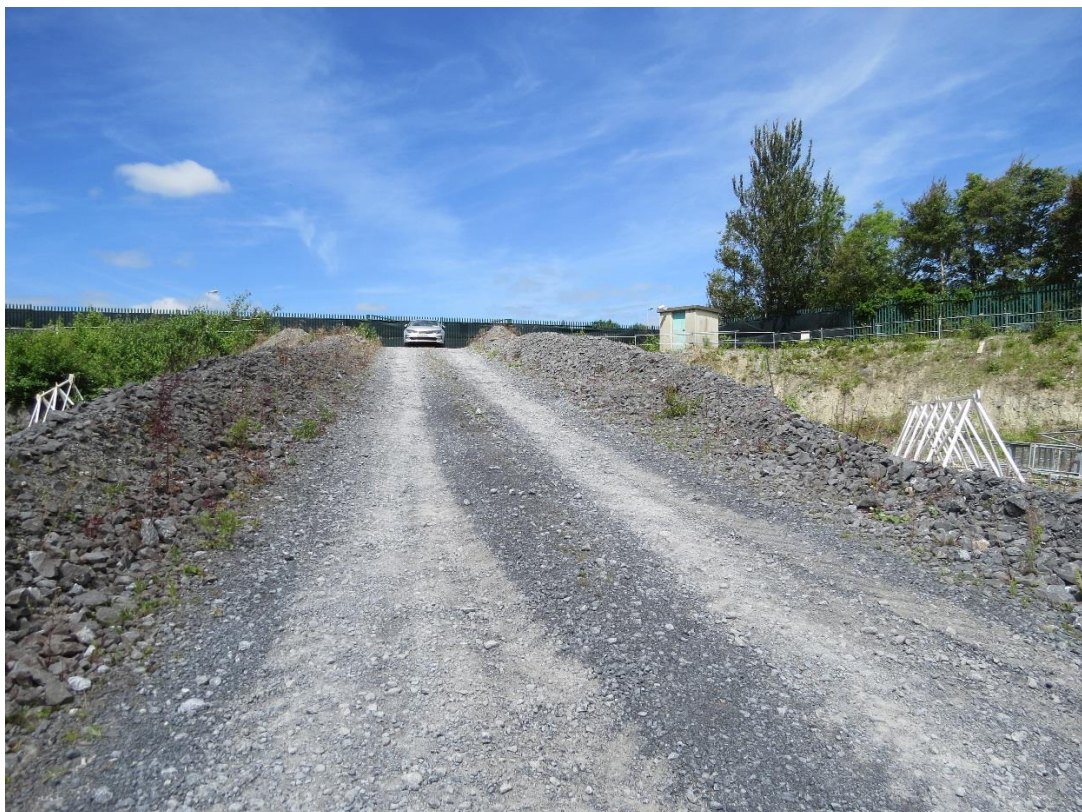
Image 2: Access ramp to basement excavation
