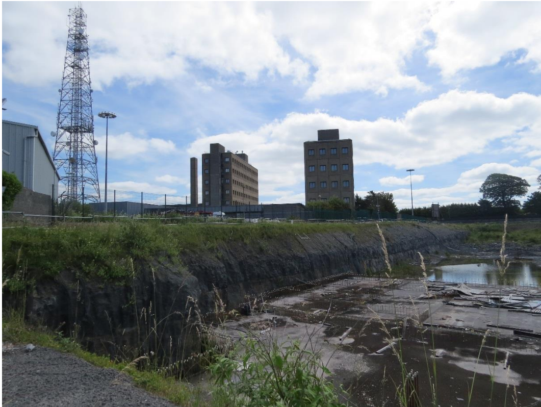
Image 3: Exposed rock in excavation on Eastern side of the site
