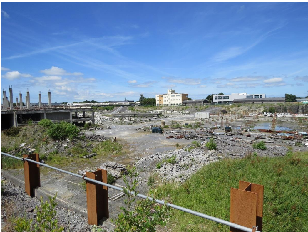
Image 6: Retaining wall on South side of basement excavation
